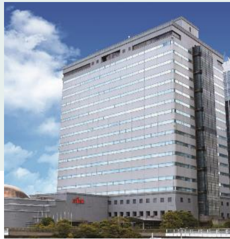
Fujitsu Makuhari Building, Chiba
