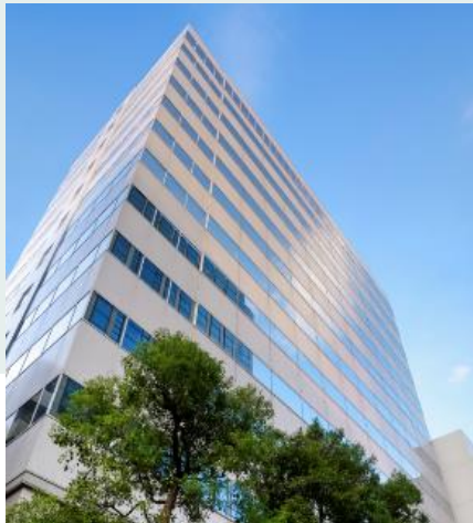
Omori Prime Building, Tokyo
